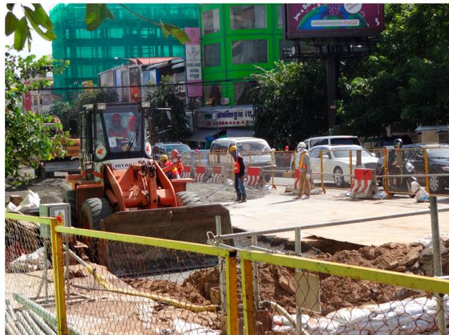
**Figure 2.** *Laying pipes. Intersection of Sihanouk and Monivong Blvds. Photo taken by author.*
